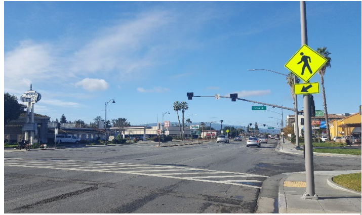
Figure 43. Pedestrian Hybrid Beacon at Morse Road / El Camino Real intersection.
