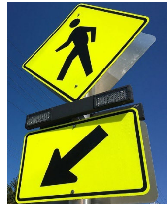
Figure 48. Rectangular Rapid Flashing Beacon (RRFB)
