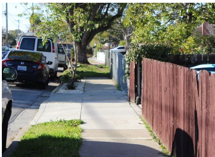
Figure 12. The sidewalk stops on Laumer Avenue and the path of travel is obstructed by a large tree
