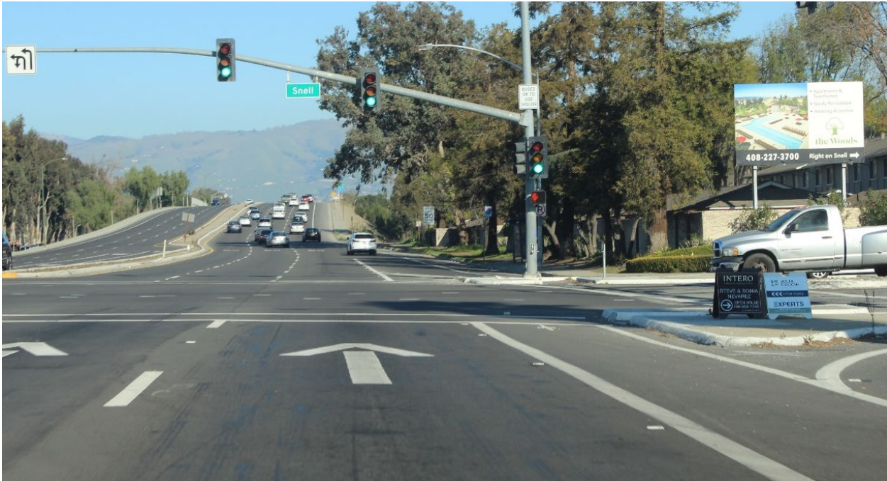
Figure 6. The Capitol Expressway/Snell intersection. People biking must merge left across right turning vehicles in the slip lane to re-enter the bicycle lane approaching the signal (not pictured). The intersection has bicycle detection, but the bicycle lane does not continue across the intersection.
