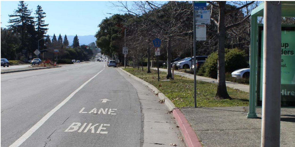
Figure 4. The bicycle lane on Page Mill Road is only marked with an inner lane marking and shares limited space with bus stops and parked cars. Parking is not allowed, but multiple cars were observed parked in the bicycle lane.
