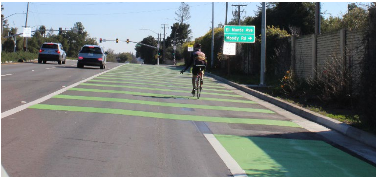
Figure 5. A person biking through the conflict markings on Foothill Expressway, approaching El Monte Avenue
