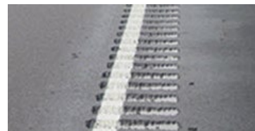
Figure 41. Longitudinal Rumble Strips and Stripes example
