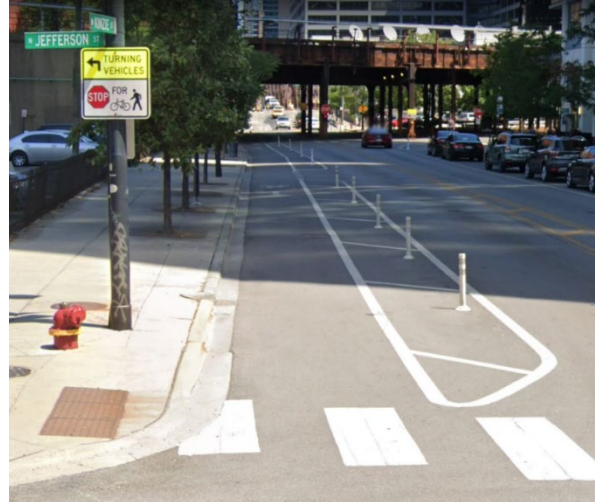
Figure 28. Vertical Buffer Alignment Placement to Accommodate Wide Bikeway Sweepers (Source: Google (Imagery - August 2019), W. Kinzie Street looking east at N. Jefferson Street)
